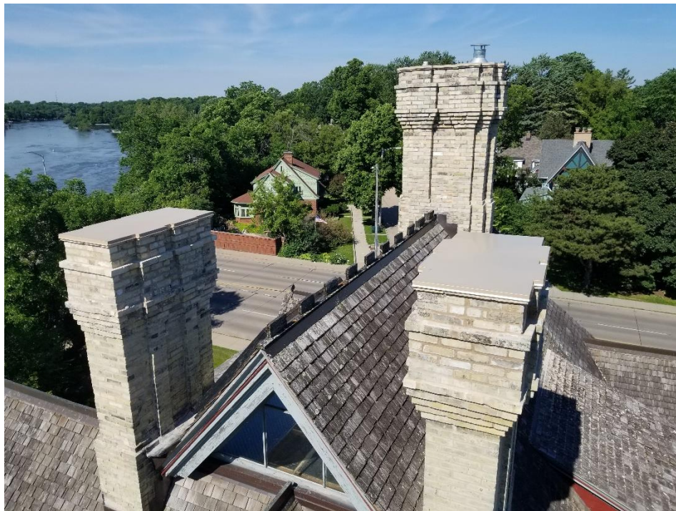
Completed Chimneys before new roof installment
