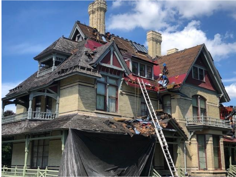
Roof Installation in 2019.
