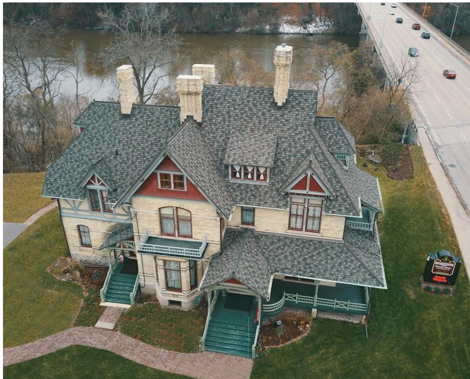
Drone View of Hearthstone showing the new long-lasting roof and completed chimneys.
